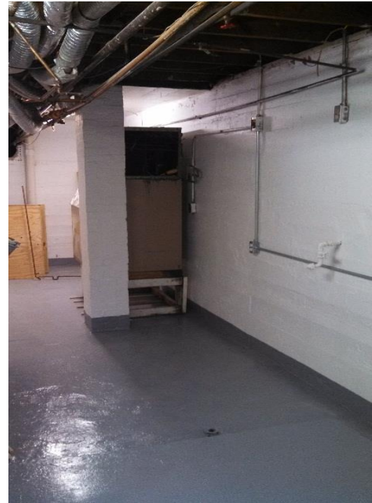
Concrete was cut for new fridges
