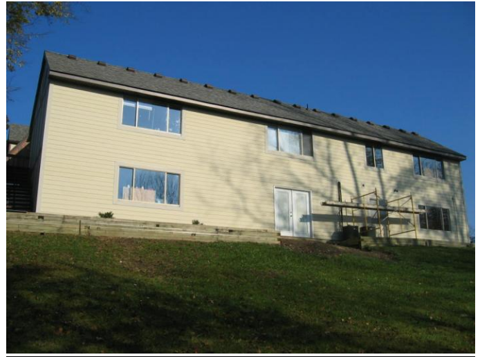
New Siding on the backside of the Addition.
